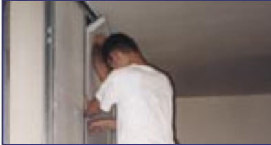
First layer of plasterboard
