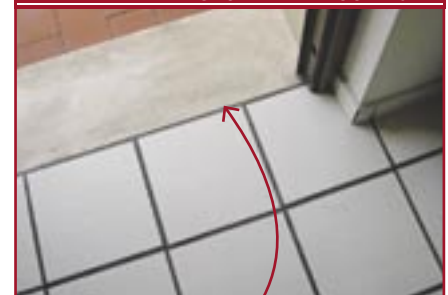
Rigid connection to the threshold -8 dB
