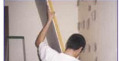
Position the SILENTGIPS slab
