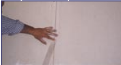
The sealing strip is positioned before the frame is laid
