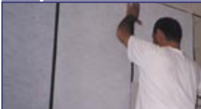
Lay and seal of plasterboard
