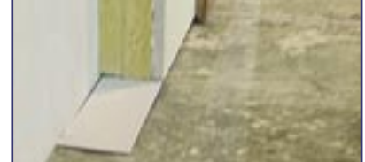
Position the sealing strip
