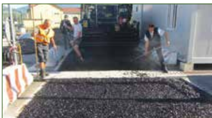
Hot laying of an open conglomerate
