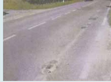
February 2014 - Inspection - 7 months after renovation without AUTOTENE ASFALTICO ANTIPUMPING
