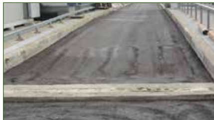
The lanes are crossed by a trench housing the services.
