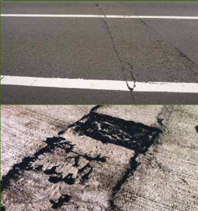
Crack-sealing operations on a mountain road in Switzerland
