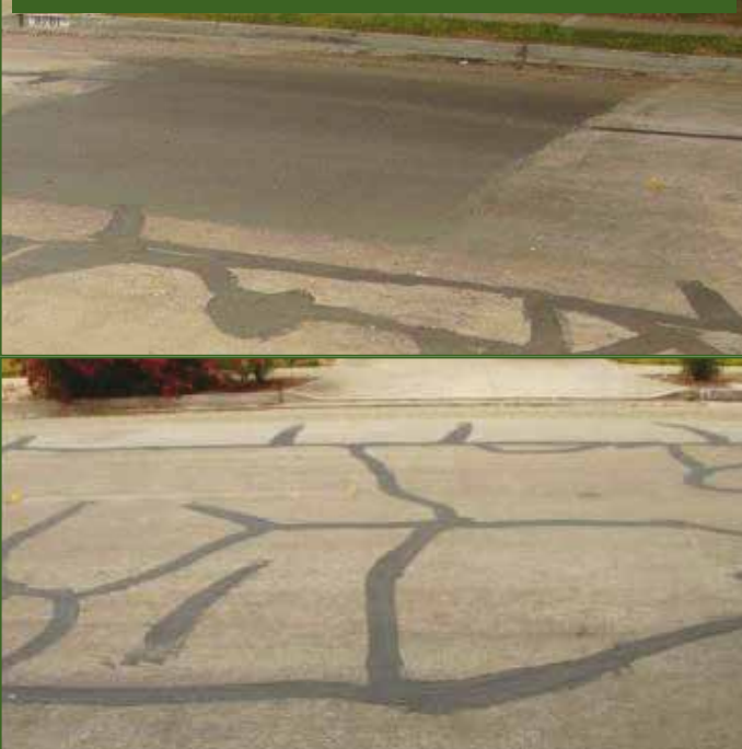
Hot sealing operations on US roads before laying an “Interlayer”
