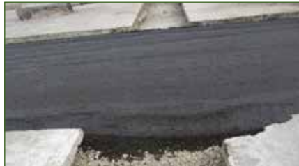
The lanes are crossed by a trench housing the services.
