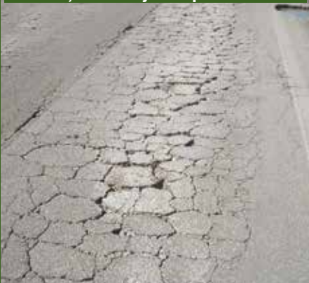
Deep crocodile cracking becoming detached in scales, structurally inadequate
