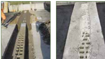
The channel is locked in place by poured concrete.
