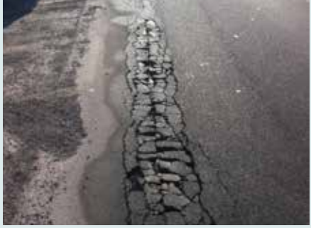
February 2013 - Existing situation
