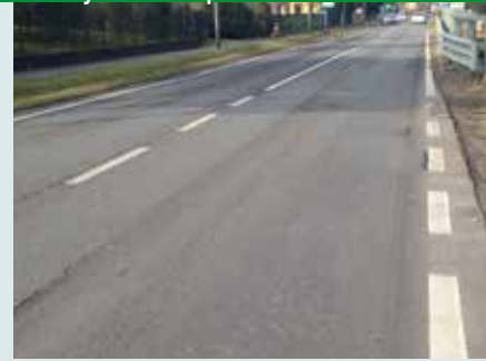
February 2017 - Inspection - 34 months after renovation with AUTOTENE ASFALTICO ANTIPUMPING
