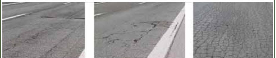
Deep crocodile cracking becoming detached in scales, structurally inadequate
