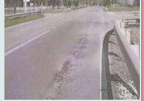
February 2014 - Inspection - 7 months after renovation without AUTOTENE ASFALTICO ANTIPUMPING
