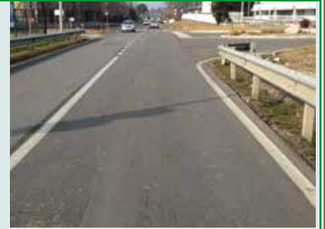
February 2017 - Inspection - 34 months after renovation with AUTOTENE ASFALTICO ANTIPUMPING
