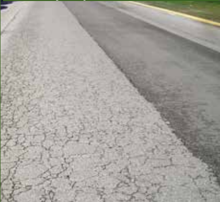
Deep crocodile cracking becoming detached in scales, structurally inadequate
