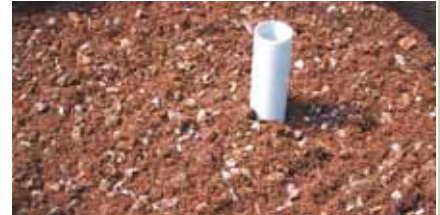
4. Laying of planting soil
