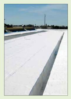
LEED - SS Credit 7.2. Heat Island Effect - Roofs Roofs painted with WHITE REFLEX reduce the "heat island" effect (differences in heat gradient between urban areas and green spaces) and minimise impact on the surrounding microclimate, as well as human and animal habitats. *Option 1*: requires roofing materials with a Solar Reflectance Index (SRI) equal to or greater than the values indicated in the table below for a minimum of 75% of the roof surface.
