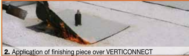
2. Application of finishing piece over VERTICONNECT
