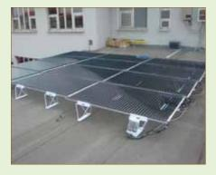
The system dysfunction was due to the bad solar reflectance values of the roof; the subsequent application of **WHITE REFLEX** paint would have demonstrated this hypothesis.
