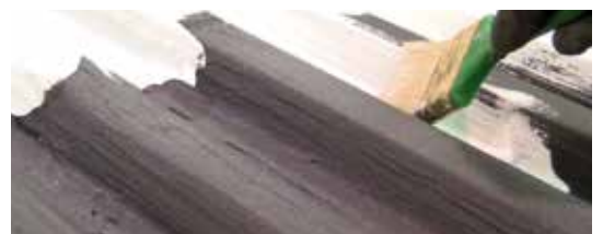
UNOLASTIC can be painted over with WHITE REFLEX reflecting paint or ELASTOLIQUID S paint
