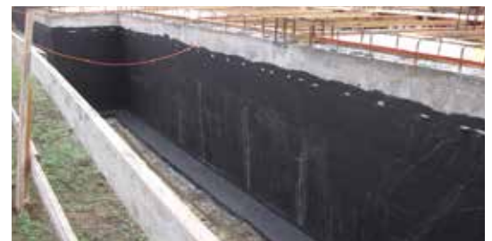
Protect the waterproofing with PROTEFON TEX or EPS panels
