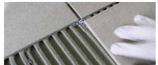
Tiles can be laid onto UNOLASTIC using adhesives C2S1
