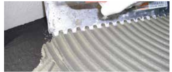
Curved tiles or shingles can be laid on UNOLASTIC fixing them straight onto mortar strips
