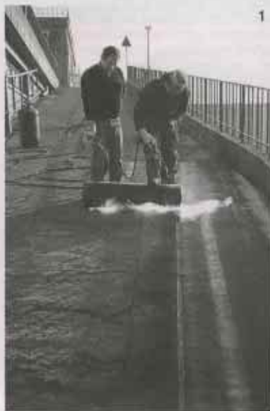
1 - Fully bonding the waterproofing on the access ramp.
